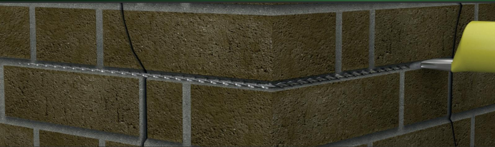
BS EN 845-1:2013 National Annex NA states that the bars need to provide an equivalent performance to the prescriptive 30mm x 5mm lateral restraint straps and the tension straps should have a declared mean tensile load capacity of at least 8kN.
